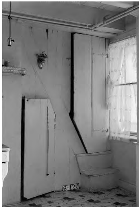
Historic American Buildings Survey, creator, and Adrian Van Houten; Nathaniel R. Ewan, photographer, July 17, 1936. Van Houten House, Totowa Avenue, Paterson, Passaic County, NJ , “Interior: Slave Stair Door”, Paterson, Passaic County, New Jersey. Documentation compiled after. Library of Congress, https://www.loc.gov/item/nj0735/ ; accessed August 8, 2017.
